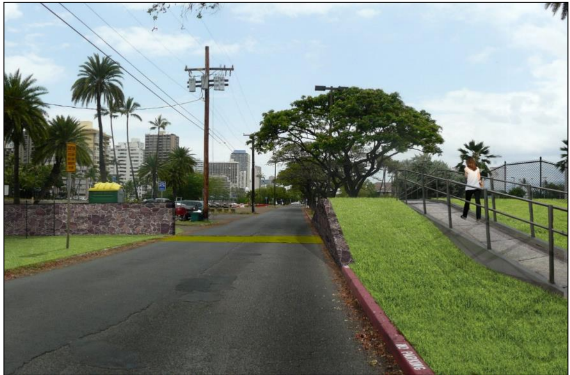
Entrance to Ala Wai Golf Course Detention
